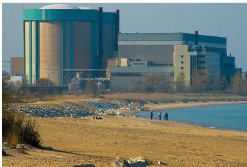
Zion Power Plant
